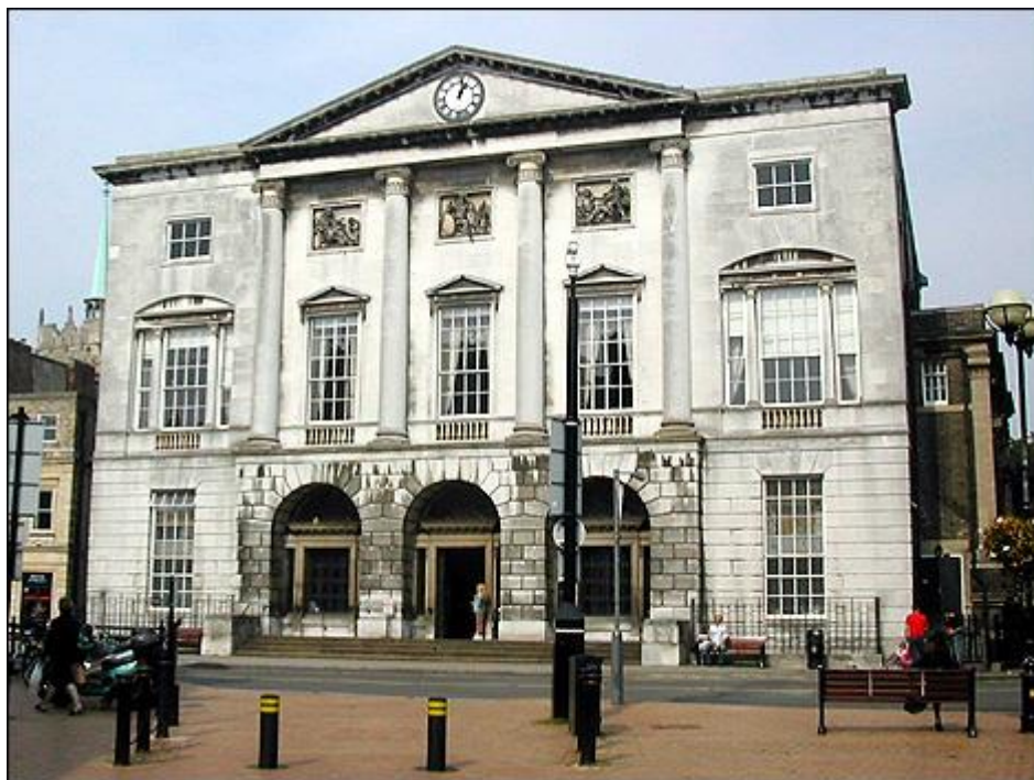
Deeper Life, Bible Church, Shire Hall, High Street, Chelmsford
