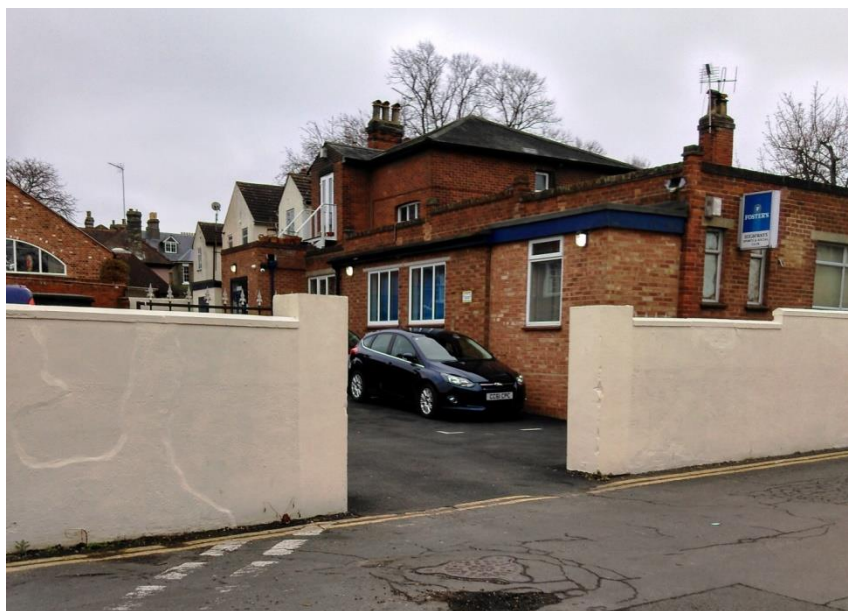
Life Church, RAD Centre, Walsingham Road, Colchester
